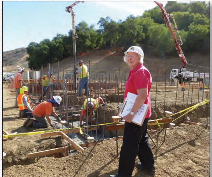
Wilma supervising the Canine Pavilion concrete pour Photo: Serenity Nichols
