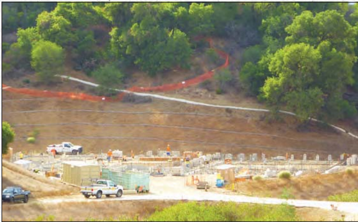
Laying block at the Canine Pavilion site Photo: Kate Horwick
